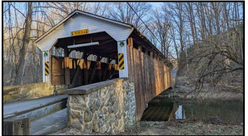
Driving south on Kings Row Road we head to **Glen Hope Covered Bridge**, the last and most southern bridge on the tour. The bridge is located only ½ mile from the Mason-Dixon Line; the border between Maryland and Pennsylvania. It is a 65-foot-long Burr truss bridge, constructed in 1889 and spans the Little Elk Creek. It has vertical planking and eave-level window openings.
